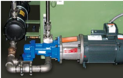
Self contained, low pressure lubrication system.
